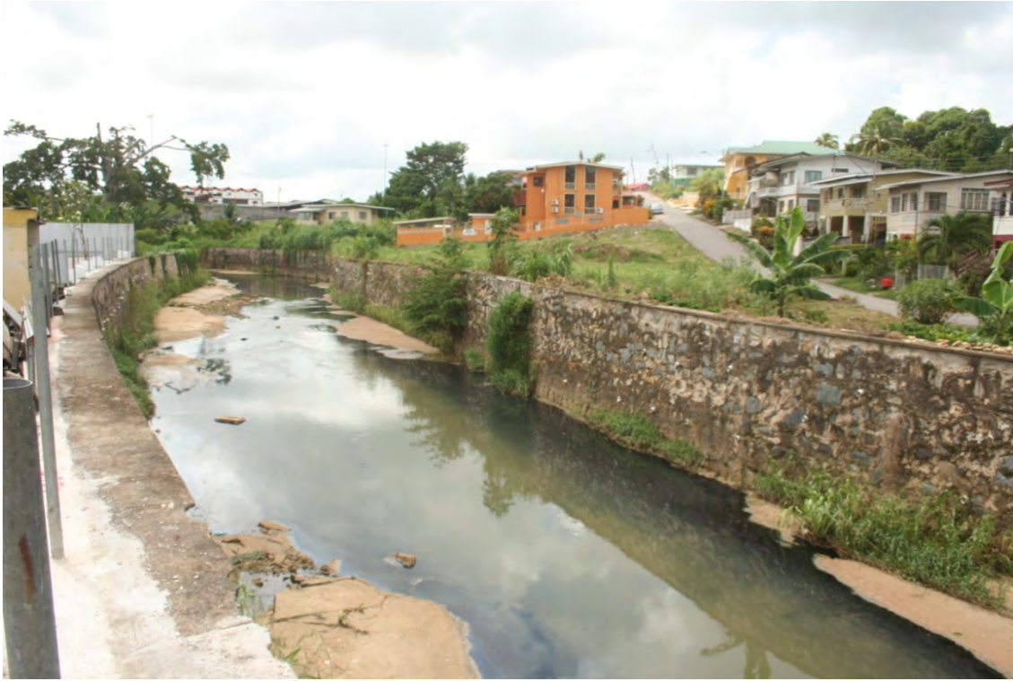
Figure 5-28 Cipero River in Concrete Channel at Grid Reference 668521mE, 1134820mN
