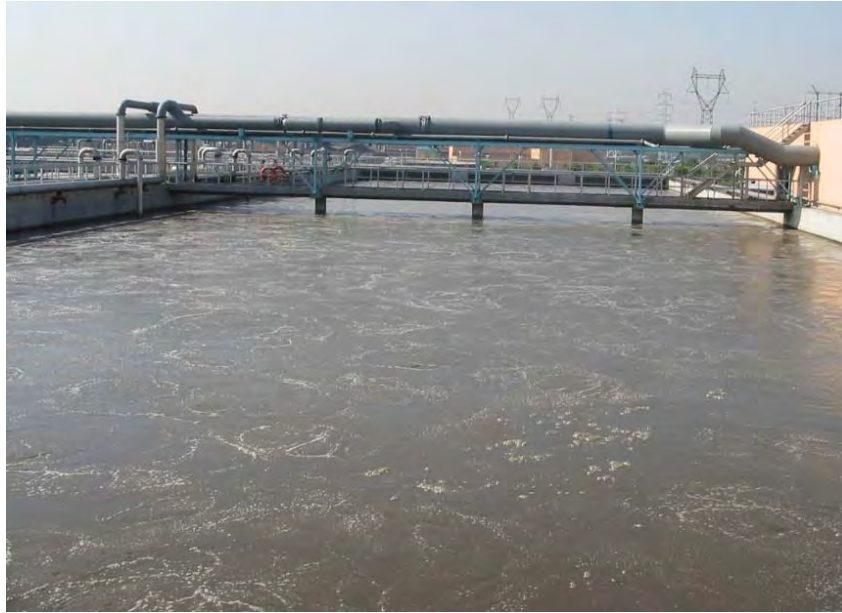
Figure 3-17 Fine Bubble Aeration Bioreactor
