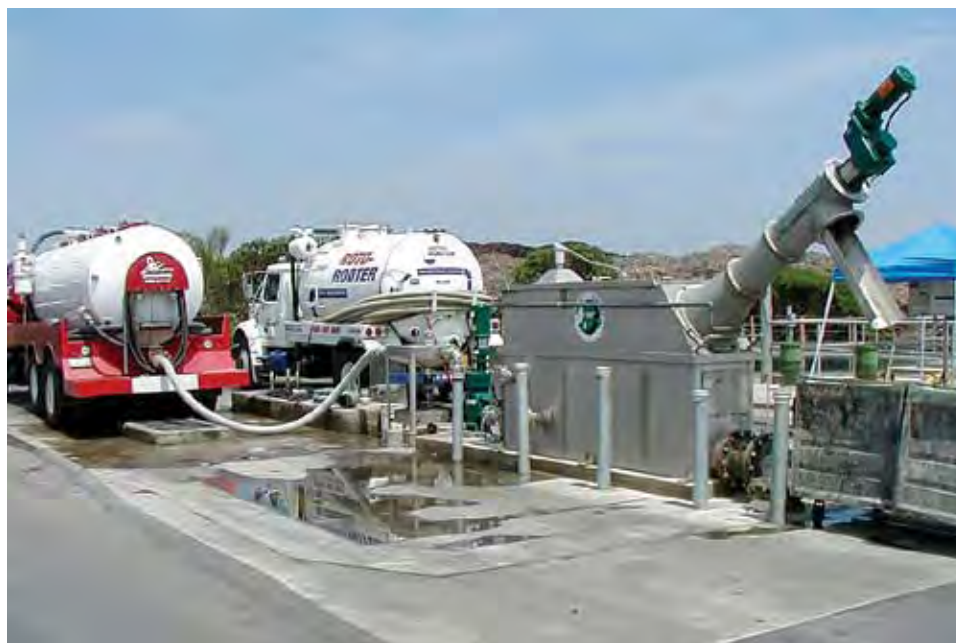
Figure 3-13 Package Septage Receiving Unit (Courtesy of JWC Environmental)
